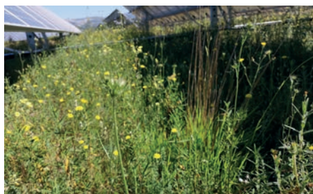
Photo 13: Photovoltaic plant in Le Castellet (83) (© Voltalia)
