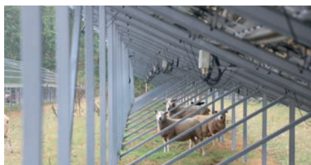
Photo 5: Sheep grazing in a photovoltaic power plant in the Allier (© E. Mortelmans)
