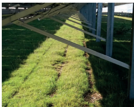
Photo 32: Fixed table on driven single-pile (© Idele)
