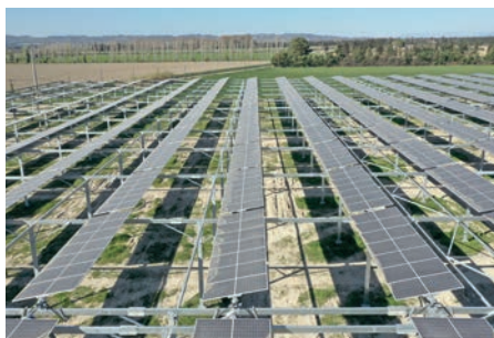
Photo 17: Photovoltaic shades at the Cabanon (© Voltalia)
