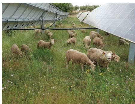
Photo 19: The 1-axis tracker control bars do not pose a problem if the animals can circulate smoothly below, as in the Canadel power station (83) (© Voltalia)
