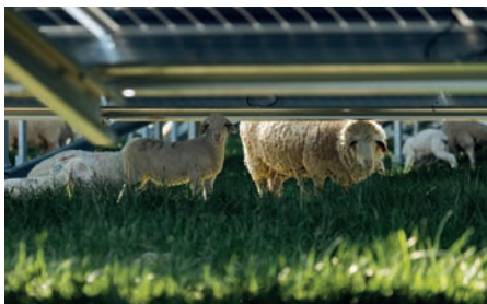
Photo 7: Sheep thatching in the shade of photovoltaic panels (© TSE)
