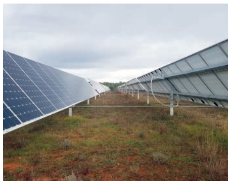
Photo 18: 1-axis tracker panel control bars that may possibly complicate co-activity with breeding depending on their height (if <80 cm from the ground) (© Idele)
