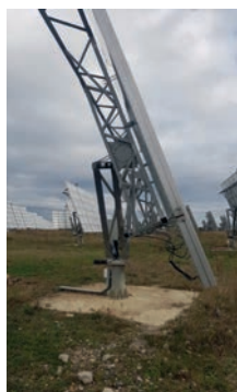
Photo 31: Single-pile double-tracker on a concrete slab (© Idele)
