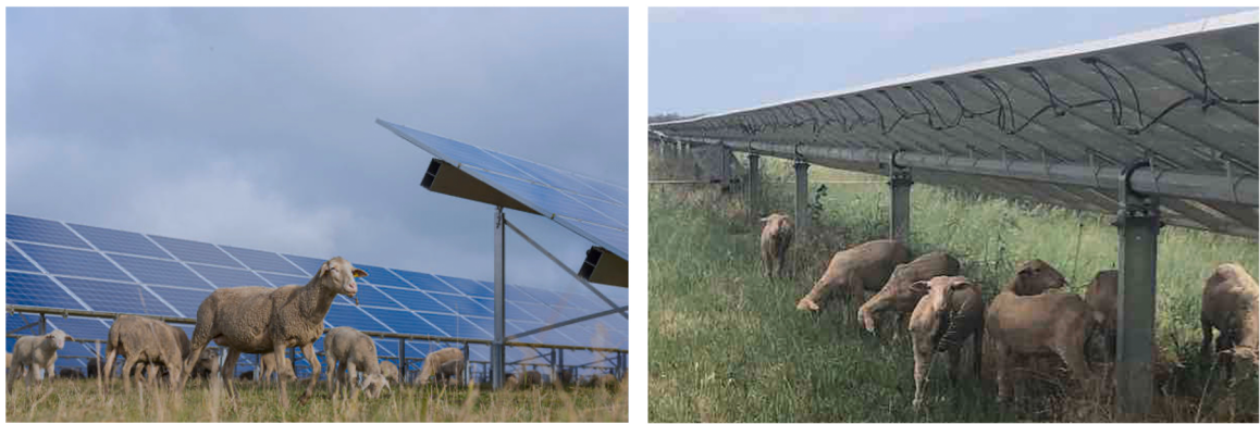
Fig. 4. Fixed-tilt (a) and single-axis tracking (b) agrivoltaic systems.
